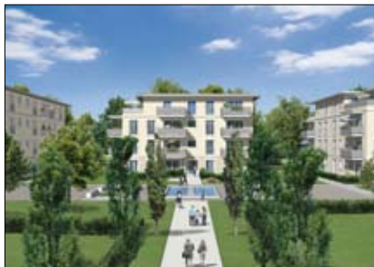
Baufeld 2 Concept Bau-Premier + SBR Arch.
